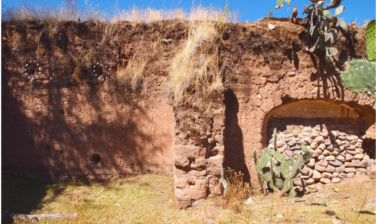
Figure 11.22: Beams for the second story of the room in which Unit O5 was located (circled in white dots).
