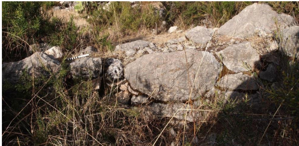
Figure 5.19: Inka-style masonry of the unusual small square structure (see Figure 5.15 for location).
