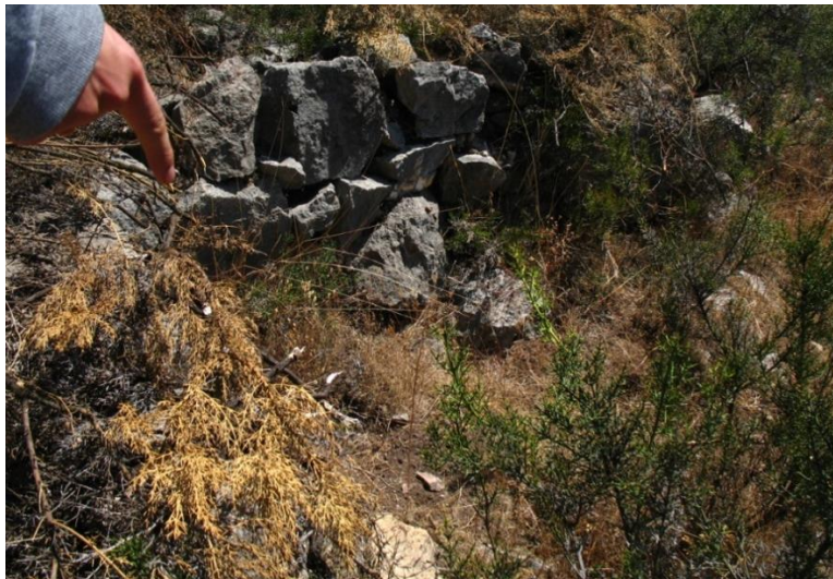
Figure 5.20: Wall of a structure that also acts as a retaining wall.
