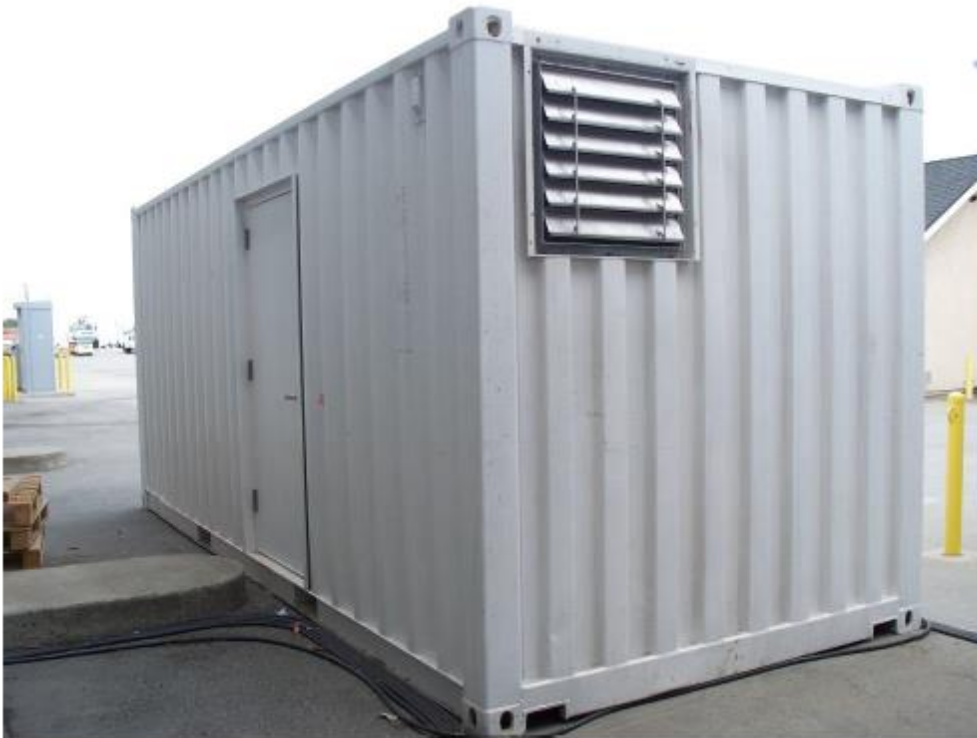
Figure 5: Battery Energy Storage System (Coleman 2013)
